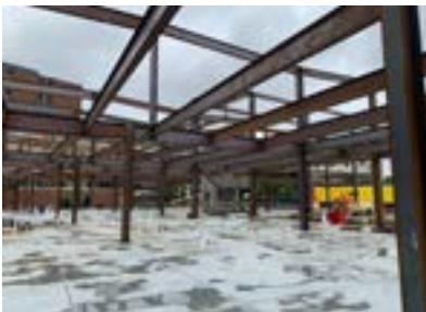
Steel framing for the new addition
