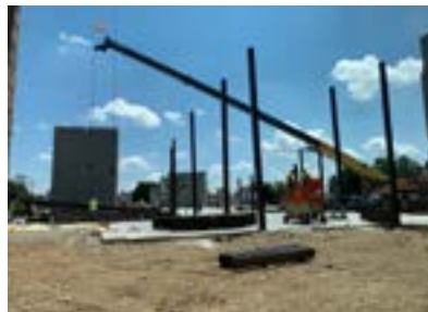
Placement of steel columns for the new addition
